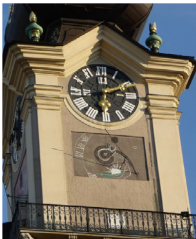
Fig. 2 Sixteenth century tower in the Parliament building in Linz, Austria. One can see the baroque helmet and in the body of the tower a mechanical clock and a sundial that are repeated in each of its facades. Sundials made using the sgraffito technique were designed by Fritz Fröhlich, a contemporary Austrian painter. Photo: Siegfried Rasper.
